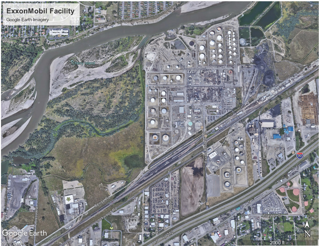
Figure 2: Google Earth representation of the Billings Refinery
